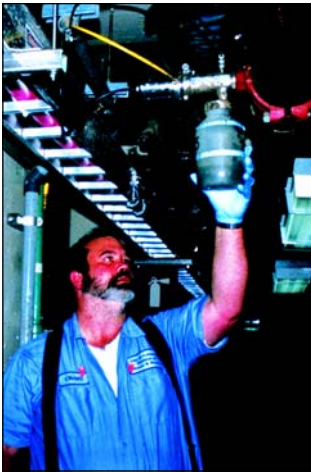
◀ Wastewater Plant Operator Craig Kidwell harvests 24-hour composite samples simply by removing and replacing the collection bottle once a day.
